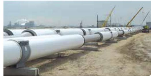
The polyisocyanurate injection systems for seamless LNG pipes' insulation before installation on site. Thanks to the fast yet precise application process under indoor controlled conditions, SPINPIPE ensures maximum quality control, insulating shell's repeatability and operators' safety. Low environmental impact (ODP = 0, GWP < 1) and full compliance to strictest cryogenic specifications make SPINPIPE the optimal solution to improve efficiency and logistics of major LNG projects.
